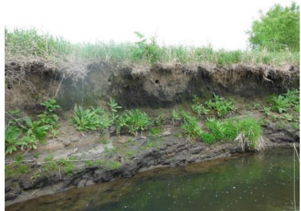
Eroding river bank
