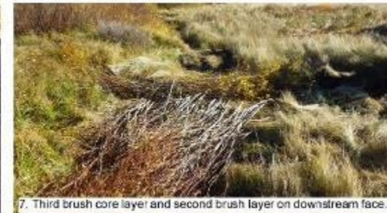
7. Third brush core layer and second brush layer on downstream face.
