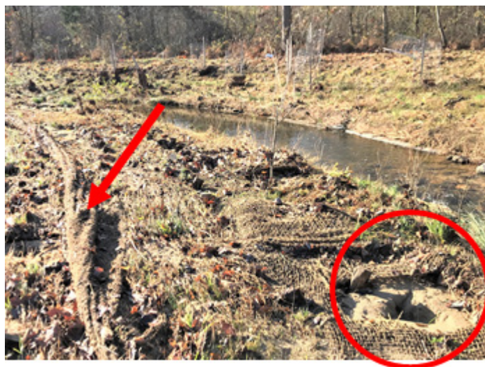
Figure 2. Floodplain erosion and fabric tear (arrow) and “potholes” (encircled) created by uprooted plant saplings following a large storm on a recently restored site. Toppled wire meshes used for planted saplings can also be seen in the background on the opposite floodplain. The photo is facing downstream, and the direction of the overbank flows is indicated by the toppled grass in the downstream direction.
