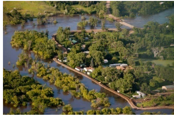
Figure 29: Levee Built around Multiple Structures
