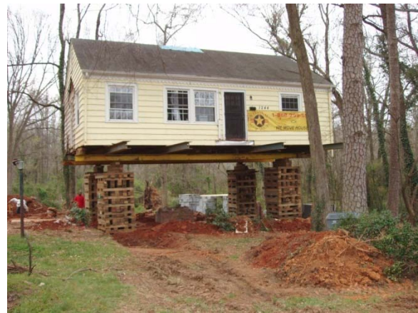
Figure 19: House During Elevation Process
