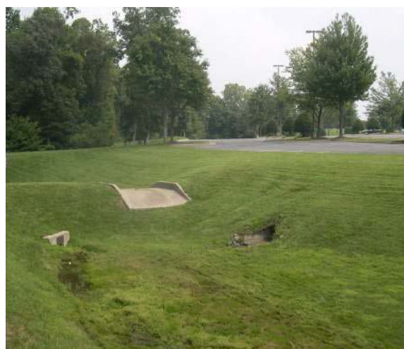
Figure 24: Example of Dry Detention Basin
