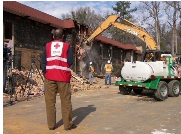
Figure 16: Example of Demolition in Progress – Cavalier Apartments
