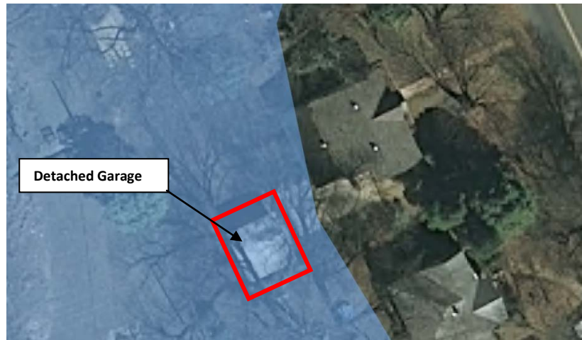
Figure 10: Example of Potential Vehicle Flooding
