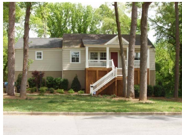
Figure 20: Completed Elevation of House
