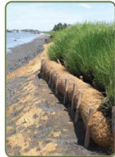
A coconut fiber log is deployed along the edge of a tidal marsh in Bivalve, New Jersey, in an effort to establish a "living-shoreline" reef that may soon protect against erosion.
