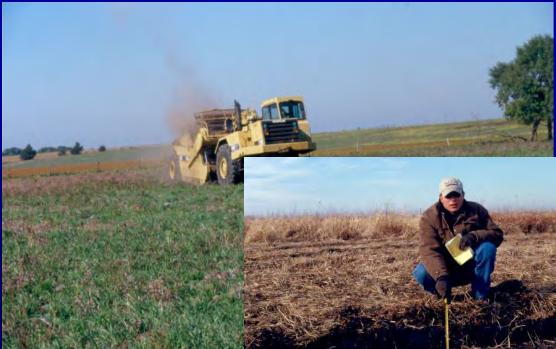
Removal of Culturally-accelerated Sediment
