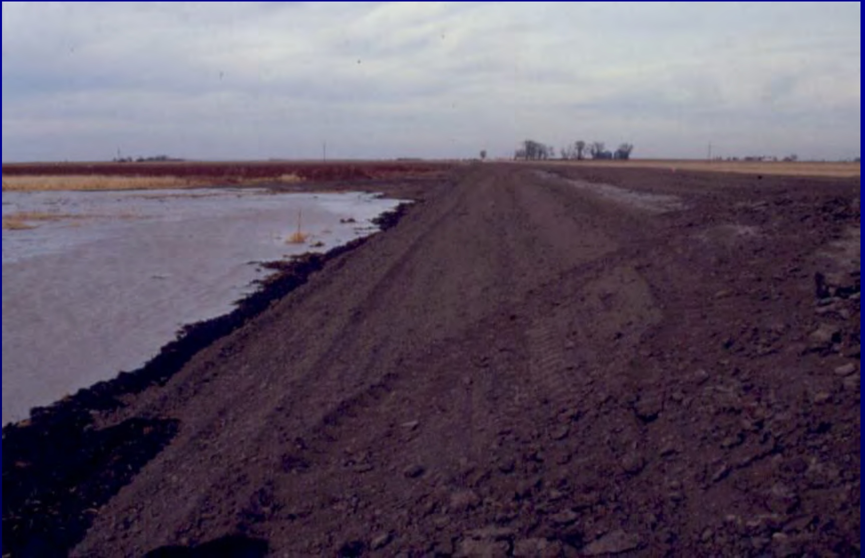
Re-contouring Road Ditches
