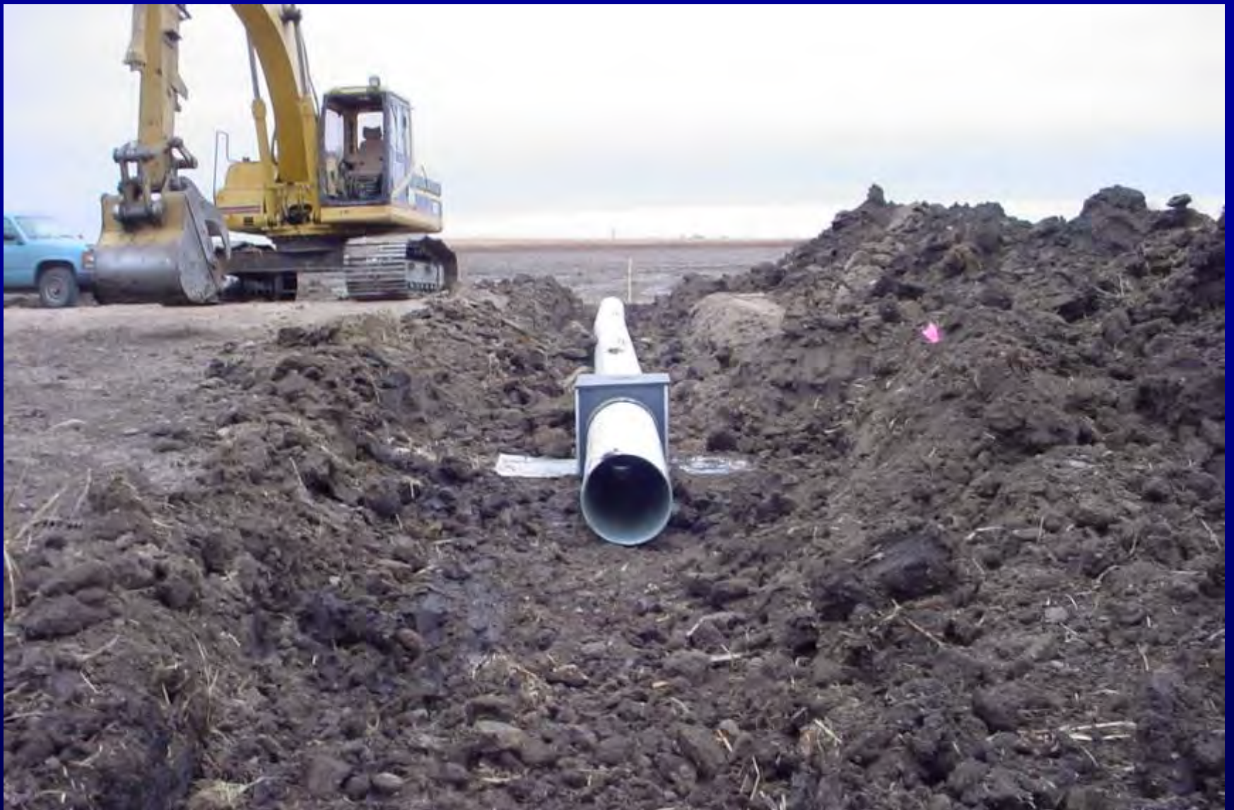
Installation of Water-control Structures
