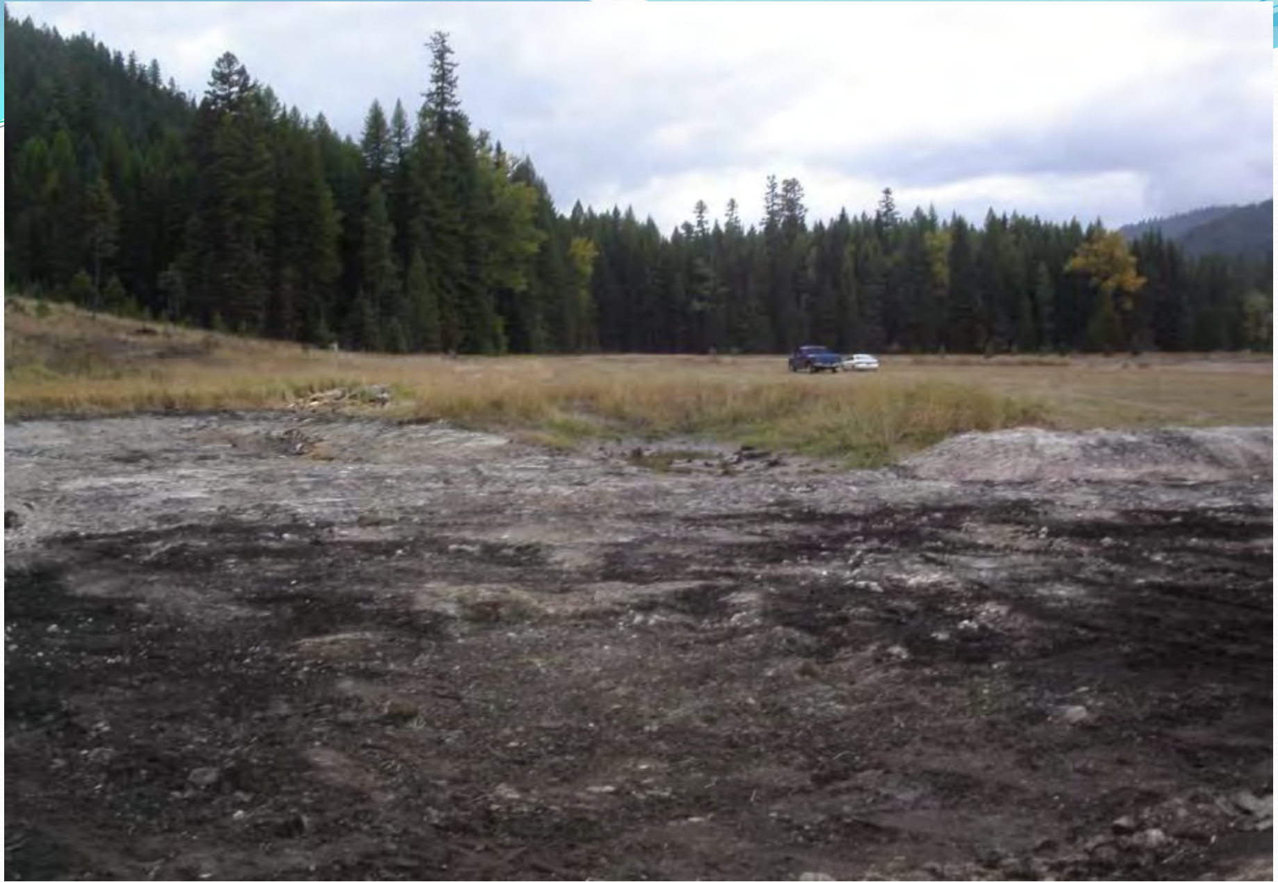
Wetland Cell excavated to reach groundwater in area exposing peat soils.
