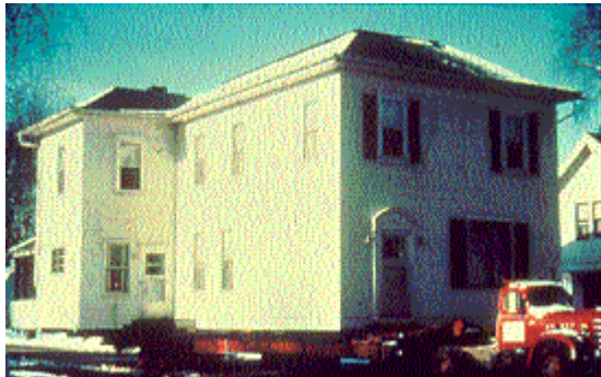
Relocation of house from wetland/floodplain areas can reduce flood losses and help restore wetland functions and values.
