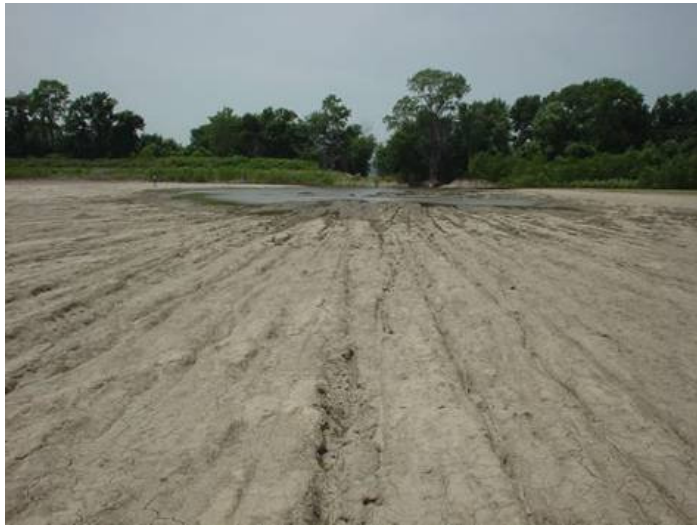
Sediment deposited at a levee breach by the Great Flood of 1993 along the Missouri river. Source: Unknown
