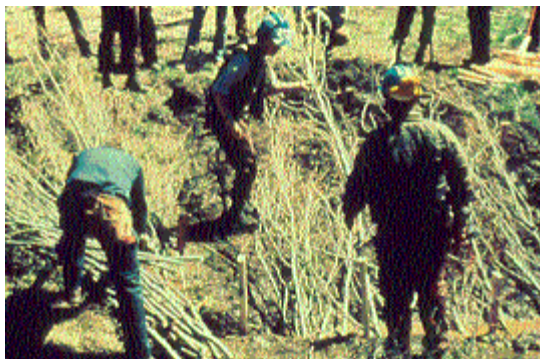
Placement of brush in stream bank bioengineering.
